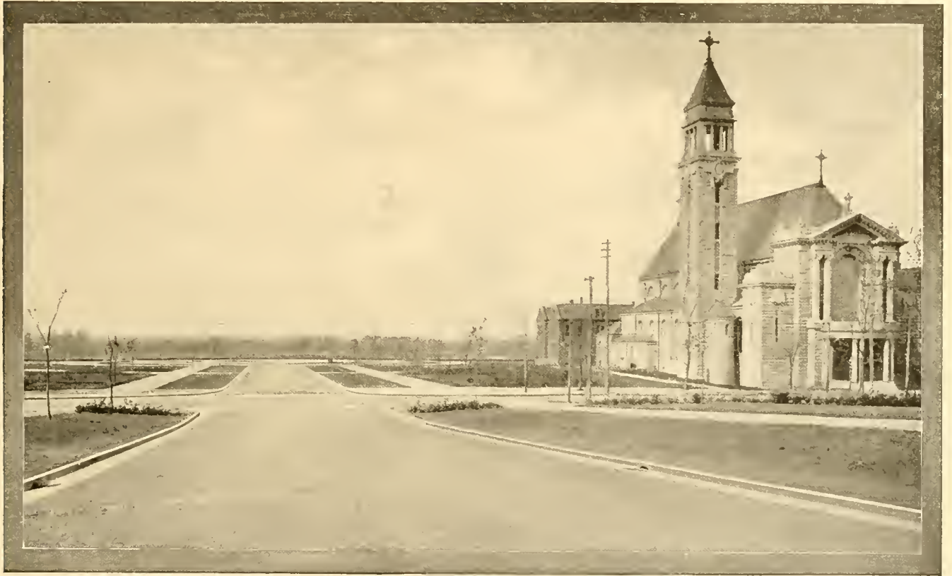
APPROACH TO WEST SIDE PARK.
